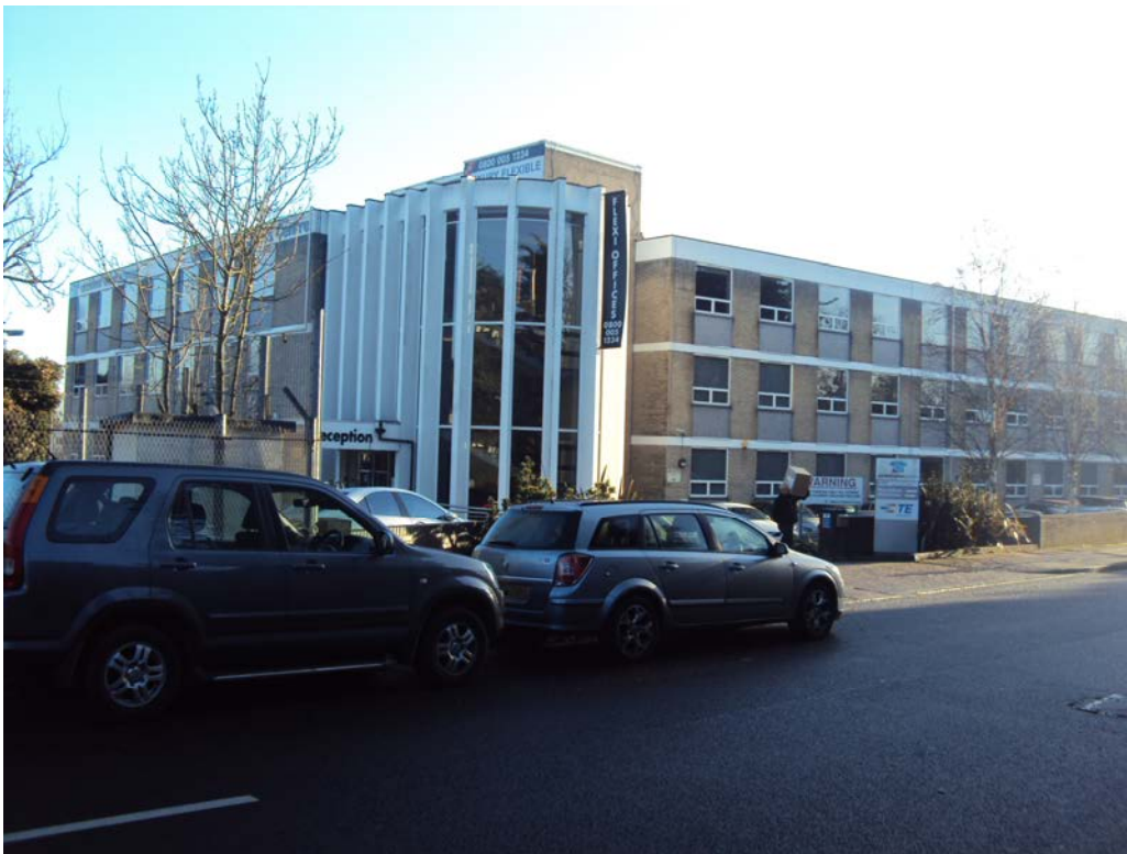
Northern elevation adjacent to London Road
