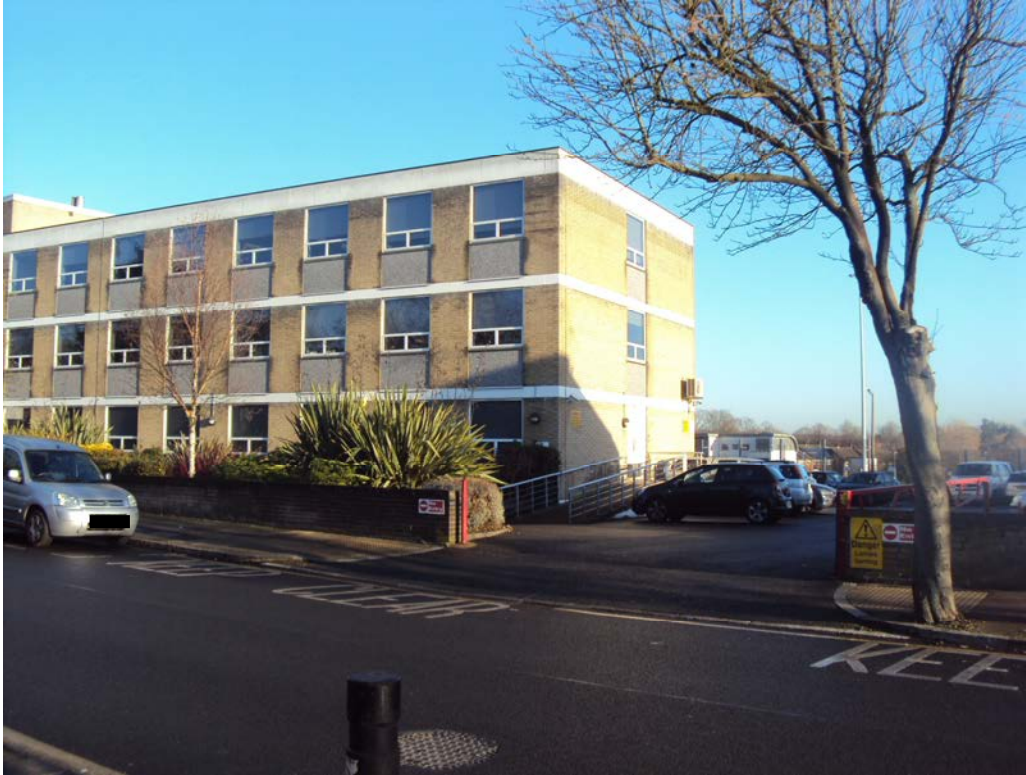
Existing Building southern end
